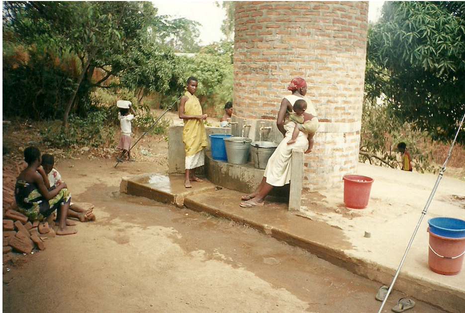
Picture 4.3: Kiosk with storage tank, KDA, Blantyre
