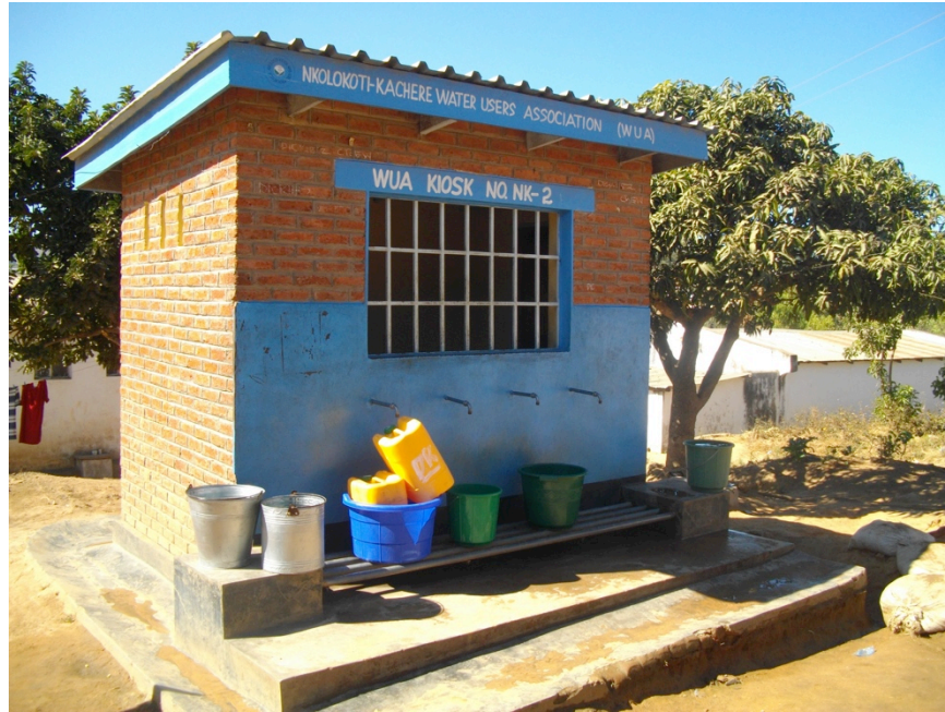
Picture 4.2: New kiosk with superstructure, Nkolokoti WUA, Blantyre
